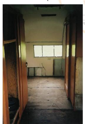
then cleaned some more. We worked all summer painting, replacing wood, replacing plexiglass with glass in the windows, checking replacing wiring, plumbing, the list goes on and on.
